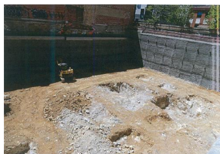
Construction site shortly before termination of original builder
