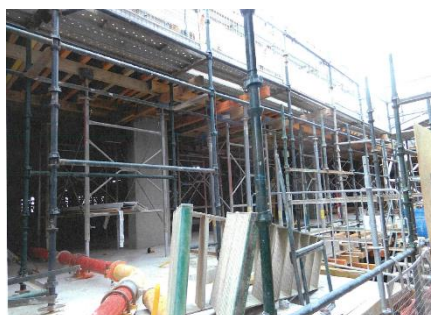
Construction site approximately four months after appointment of new builder
